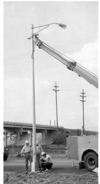
Completing installation of streetlight standard.
