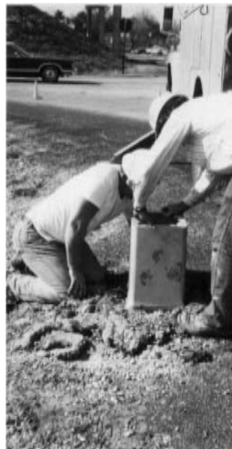
Base of streetlight standard is attached to the foundation.
