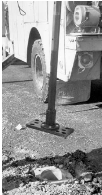
Kelly bar and drive tool assembly are removed.
